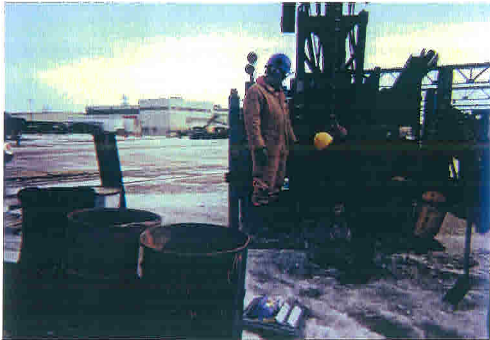
Figure 2. Worker standing next to forklift in snowy area.
